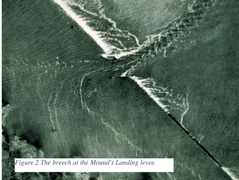
*Figure 2 The breach at the Mound's Landing levee.*
