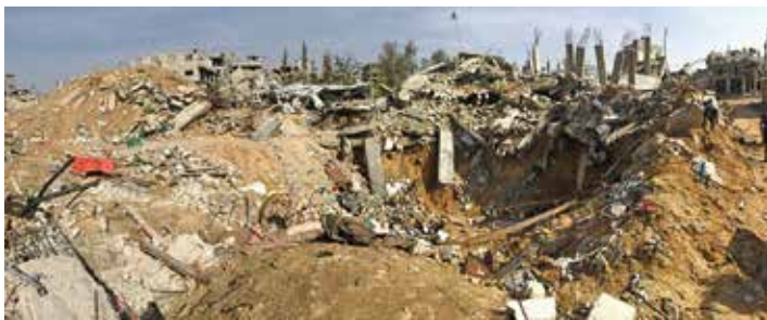
Destroyed residential area of Shejaayea.
