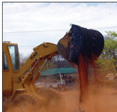
A bucket is used by an FEL to deposit soil into the sifter.
