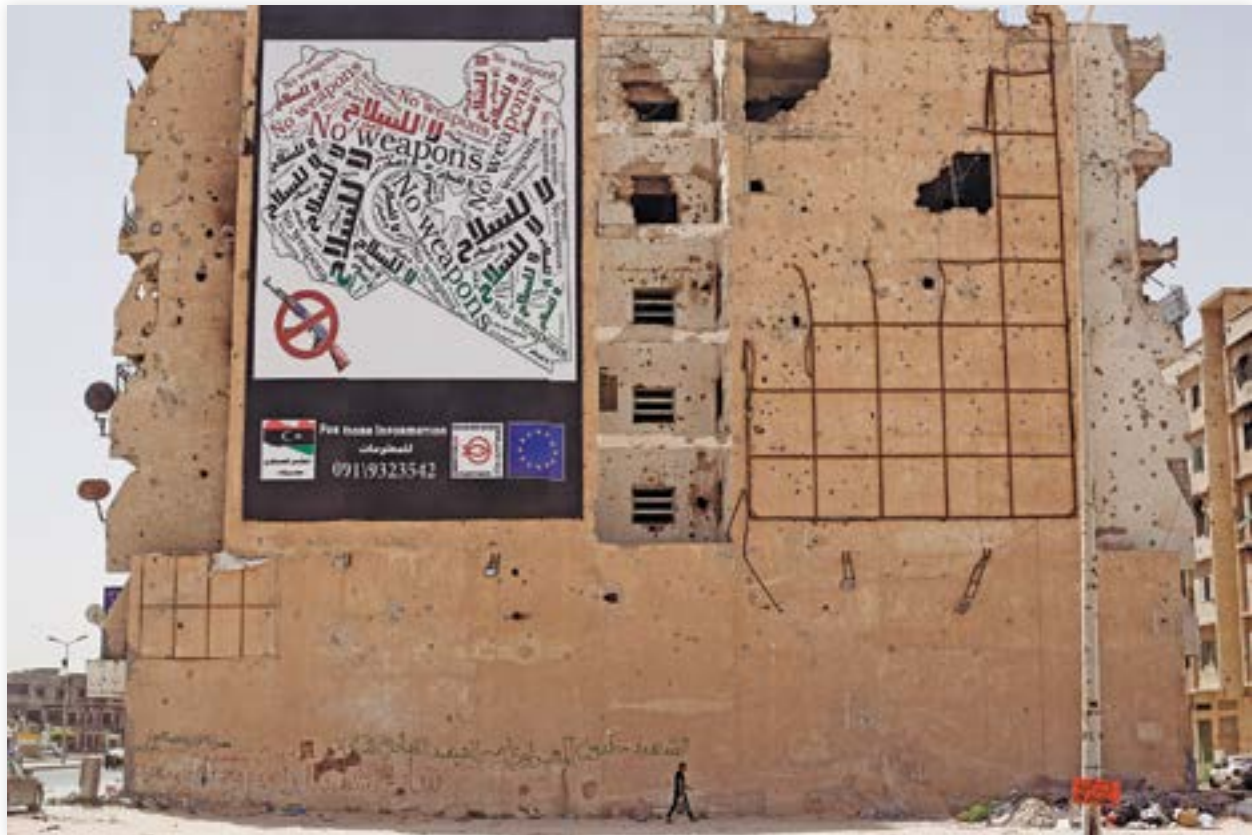
A large sign campaigning for a reduction in armed violence hangs on the side of a damaged building in Libya. The campaign was funded by DCA to inform Libyans on the dangers of weapons. Photo courtesy of Tobias Selsnæs Markussen.
