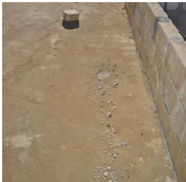
Image 9 (top) and 10 (bottom). M Series DPICM impact patterns on a roof in southern Lebanon from the 2006 conflict, showing the central hole (since filled with cement) made by the shaped charge. Note the relatively neat scarring from the pre-scoured fragmentation jacket of the DPICM. Photos courtesy of the author.
