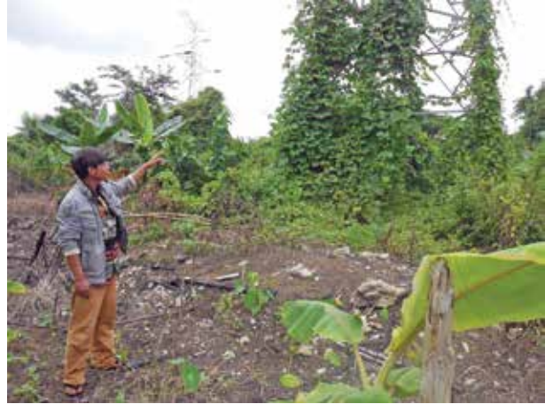
A key informant shows the hazardous area around an electricity pylon. No fences or signs warn the local population, Pa Ra Hi Ta village, Loikaw township, Kayah State.
