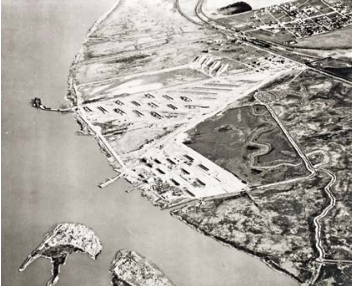
Looking eastward in early 1944, the town of Port Chicago is in the upper right corner. Utility and personnel piers extend toward the two sections of Seal Island in the lower left corner. The munitions-loading pier curves to the left beyond 20-odd revetments. Marshy tidal zones separate the munitions pier from barracks near the personnel pier and near the town.
