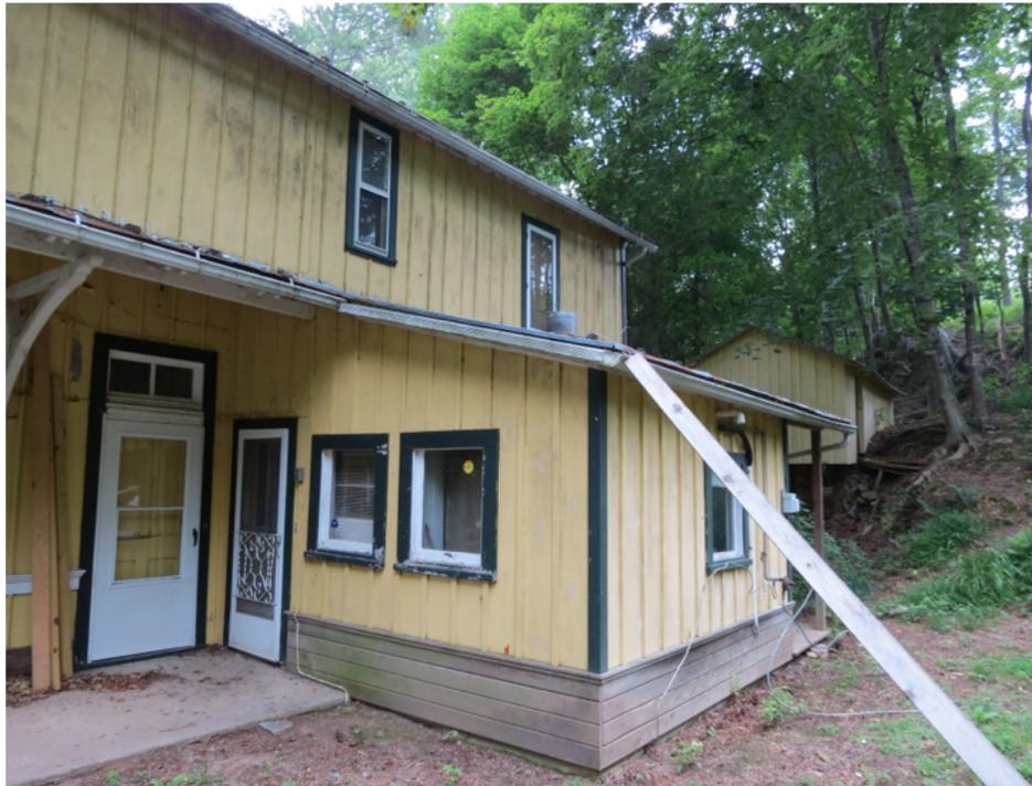
Figure 19. Areas of dirt and mildew can be seen on the exterior of the building
