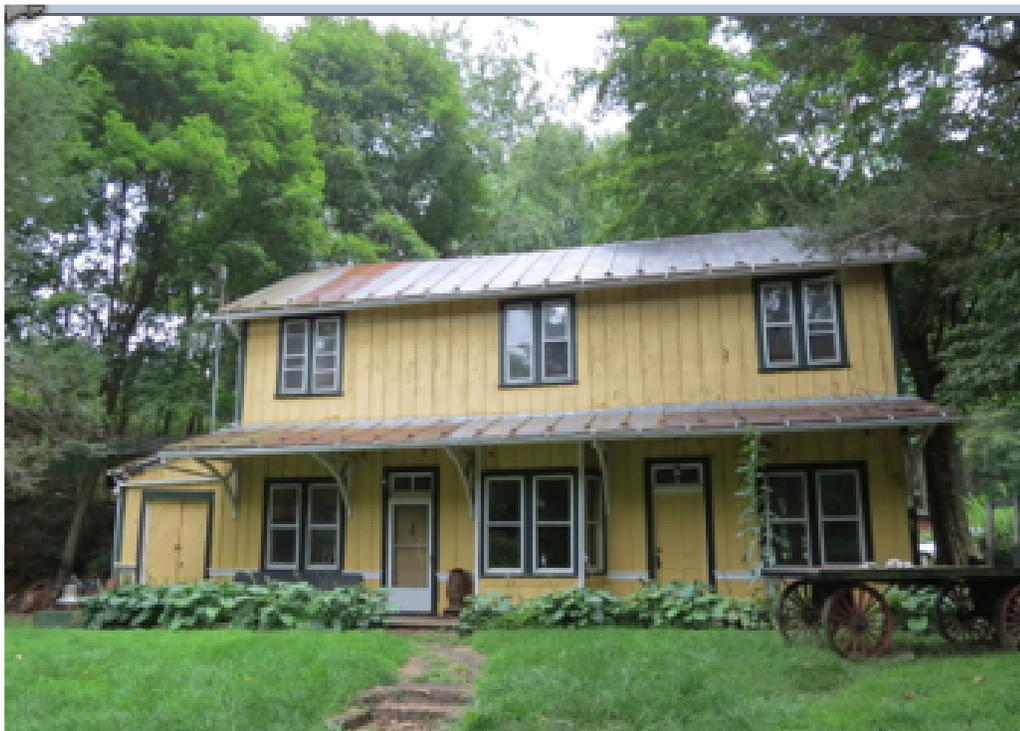
Figure 5. Northern elevation showing the building's metal roof (with snowguards), board and batten siding, green trim, and white ornamentation
