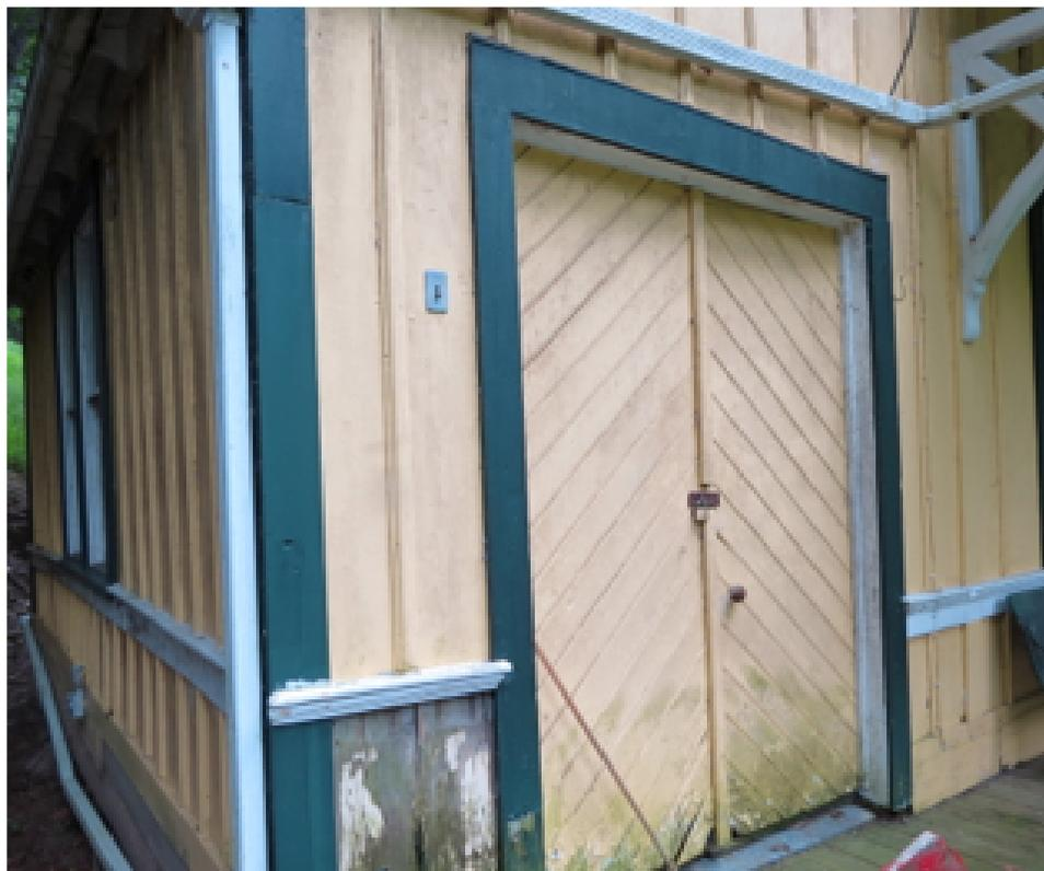
Figure 6. Two diagonal batten doors lead into the storage shed.
