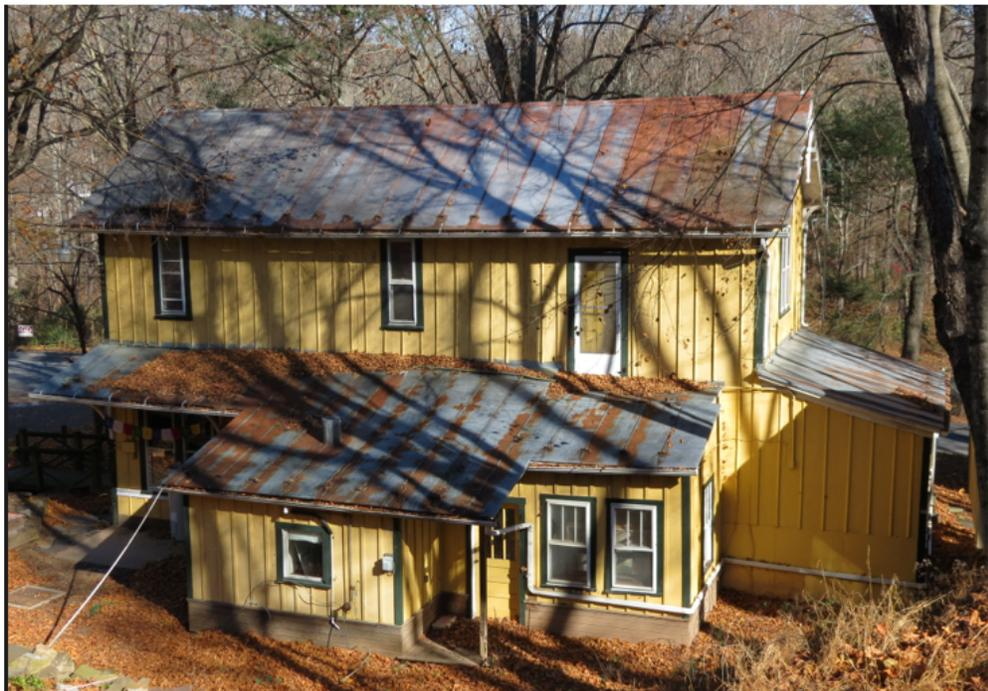
Figure 18. Southern elevation of depot showing the excessive rusting of the roof
