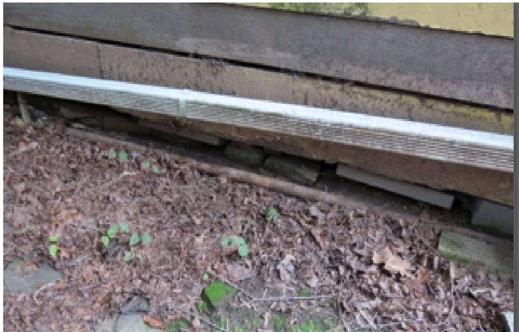
Figure 4. Rotting wood reveals elements of the foundation
