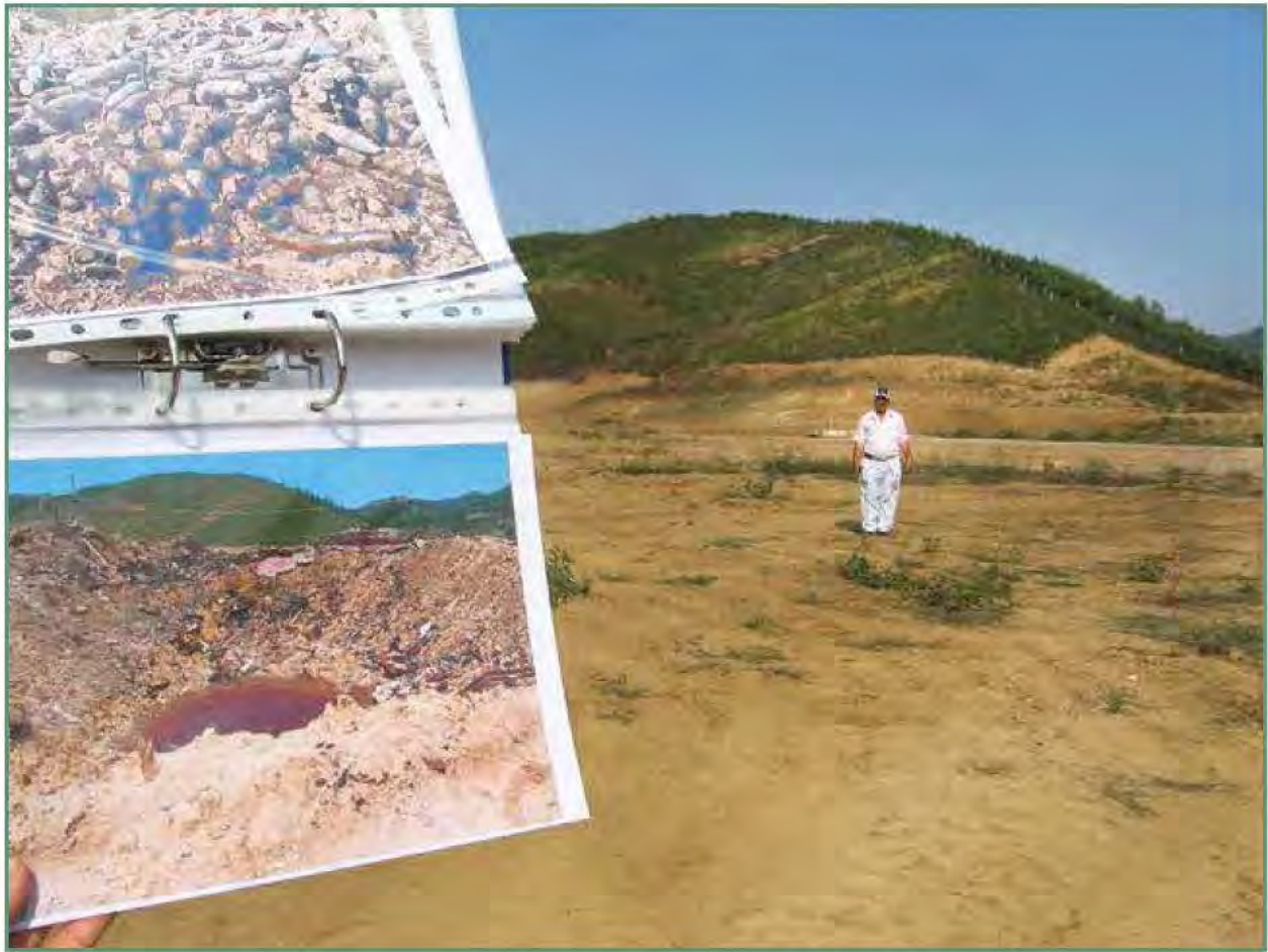
Before and after shot at the Gërdec UXO remediation site in Albania. The giant craters left by the catastrophic explosions during the 2008 disaster have since been carefully cleared of UXO and filled in thanks to U.S. assistance. Photo courtesy of John Stevens, PM/WRA, U.S. Dept. of State.
