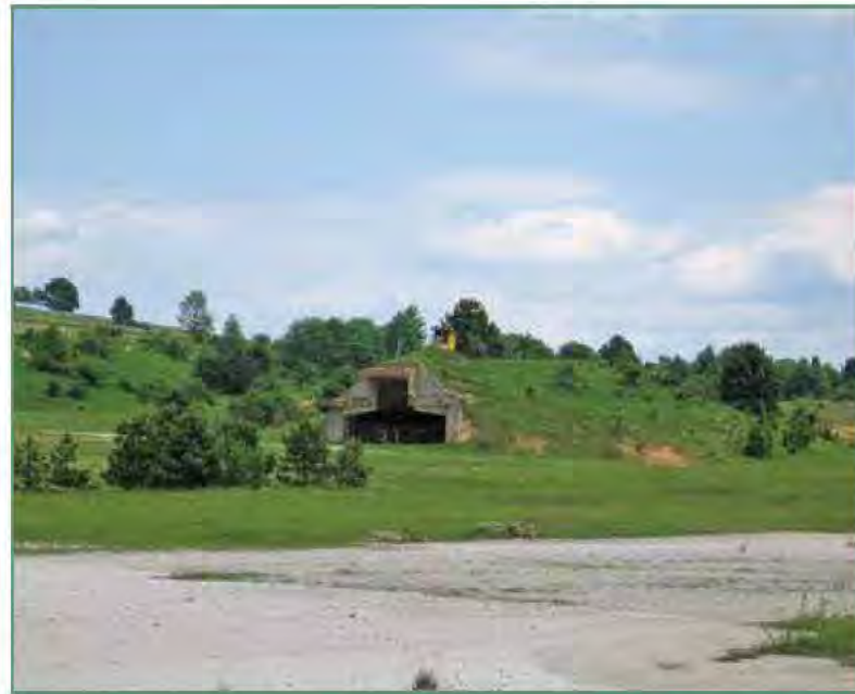
During NATO airstrikes on the Federal Republic of Yugoslavia in 1999 that led to the withdrawal of Yugoslav forces from Kosovo, the runway and military aircraft shelters at the Ponikve airfield were bombed. Now that the Ponikve airfield will be used for commercial airline flights to facilitate tourism to Serbia's scenic western region, PM/WRA helped to fund a technical survey for unexploded bombs in the grassy area between the runway and the shelters, such as the one pictured above. No unexploded bombs were discovered in areas examined with PM/WRA's funds.
