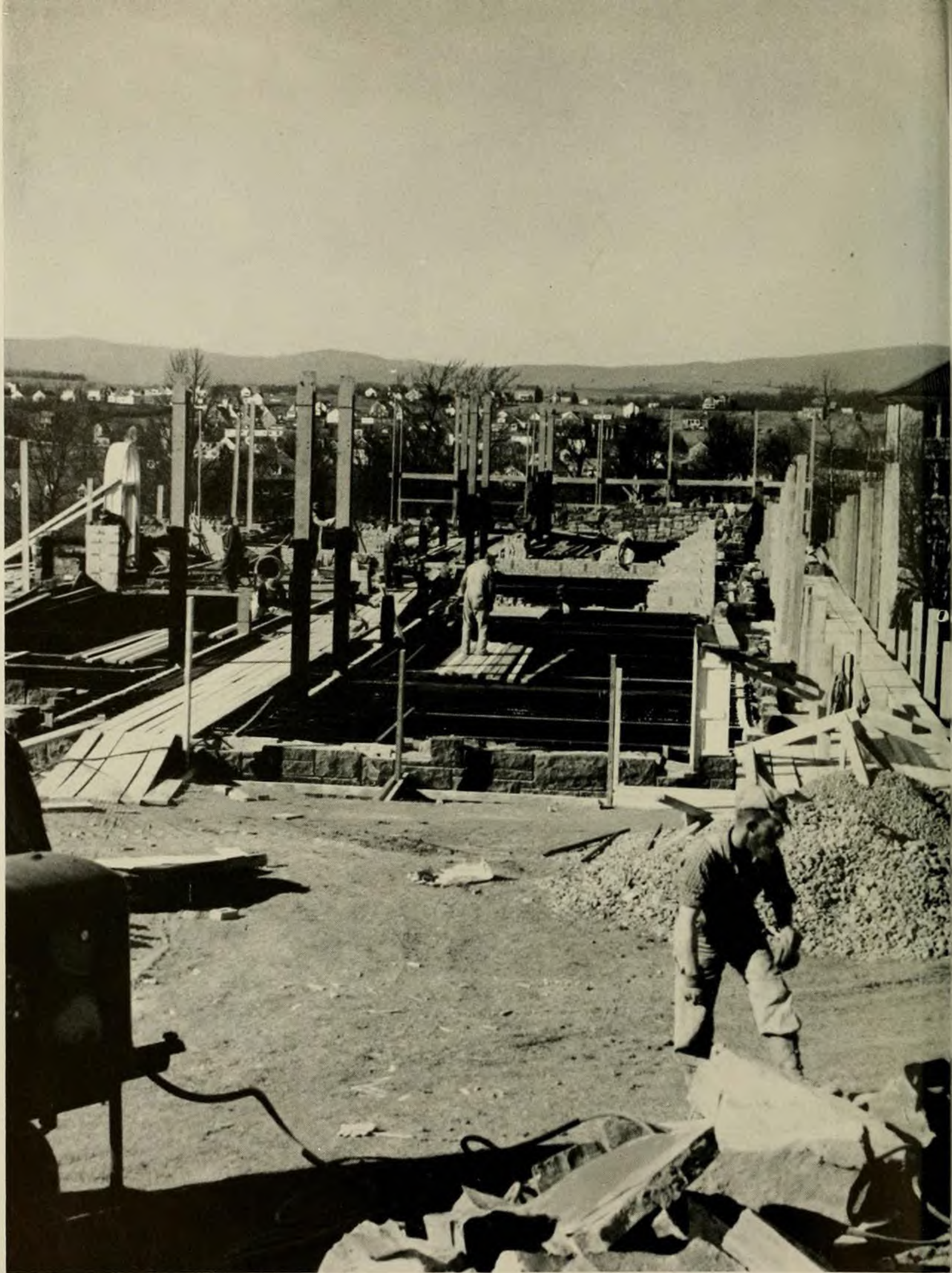
LAYING THE FOUNDATION FOR LOGAN HALL
