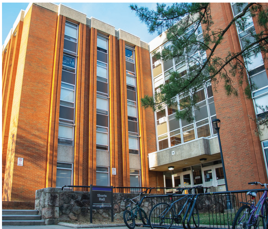
Construction of Shorts Hall was completed in 1968. Valerie Chenault / The Breeze
