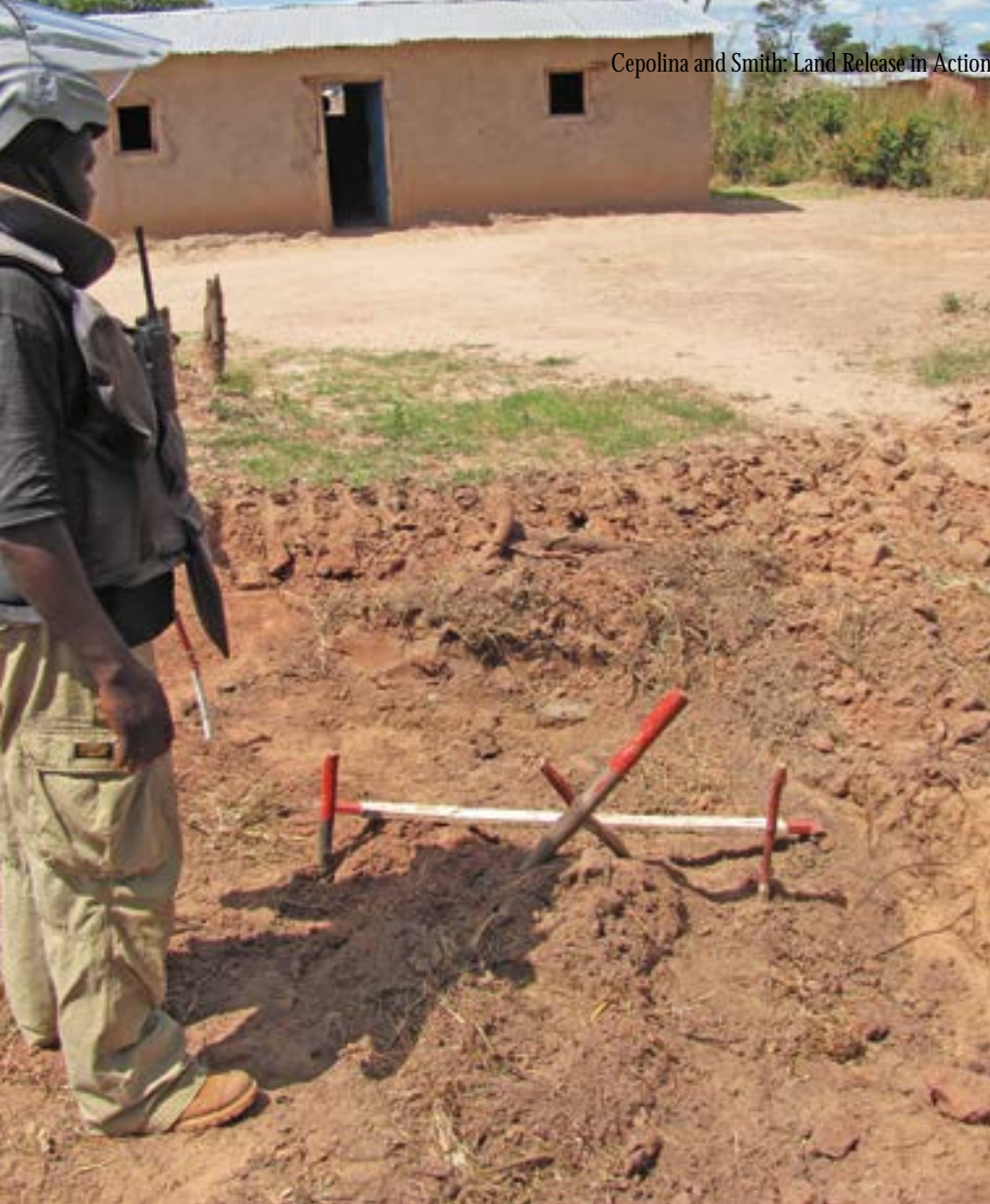
This manual deminer found an AT mine booby-trapped with a small AP mine during TS after the soil was softened by a machine.
