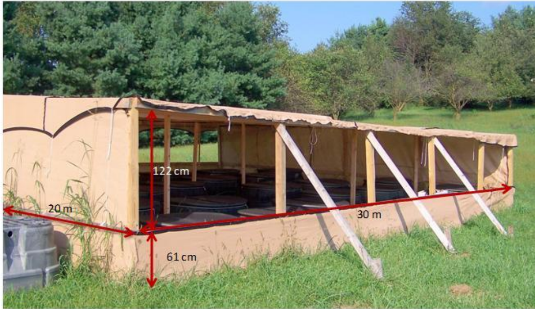
Figure 3: Photograph of shade canopy structure. Shade cloth was secured around the outer perimeter, on the top, and on the east and west sides of the structure.
