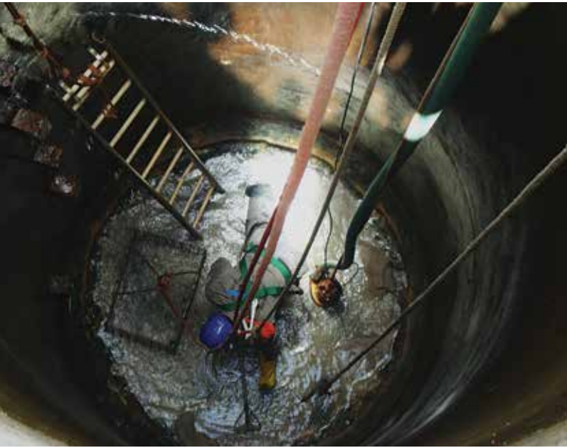
The deminer searches for hazardous objects in the well. All photos courtesy of FSD.
