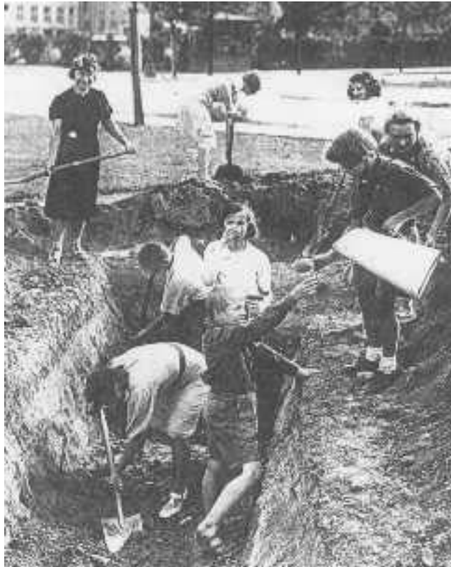
Polish civilians digging defensive ditches during the siege. 16
