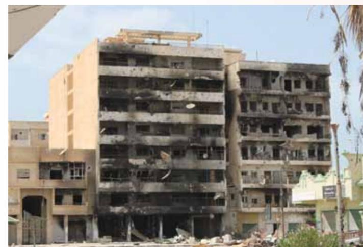
An area showing more moderate damage. Much of the damage to this building is from fires rather than from the blast or fragmentation effects of UXO. A small number of UXO items were found in the buildings pictured.
