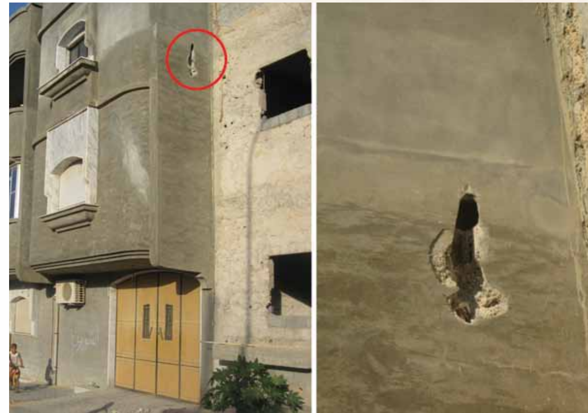
Can you spot the UXO? This neighborhood has no readily identifiable fragmentation or battle damage, yet apparently has UXO, as reported to DCA by a neighbor. It is unlikely to have been spotted by BAC.
