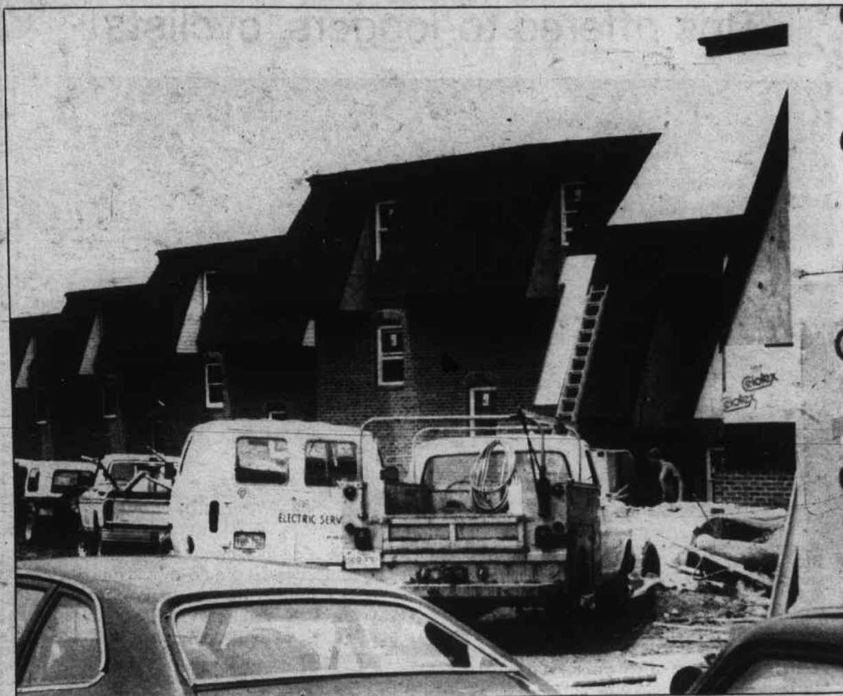
College Station, Harrisonburg's newest apartment complex, is the first local residential community to have a water sprinkler system installed for fire protection.
