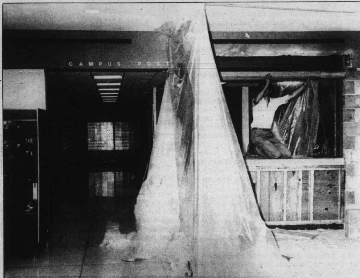
A construction worker places a beam in what will be the post office window. The extension of the window into the lobby will make room for additional mailboxes.
