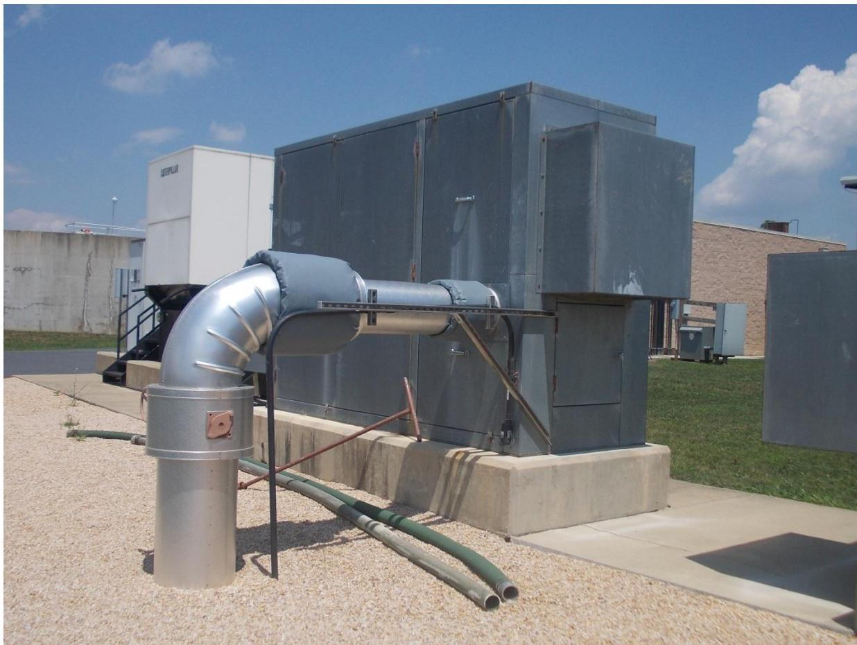
Figure 4.3 One of the three multi-stage Hibon Centrifugal blowers
