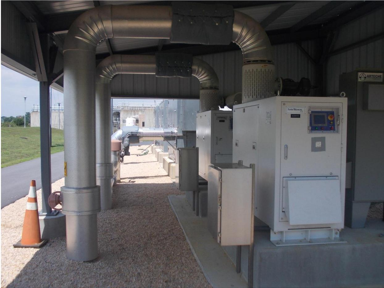
Figure 4.4 The two active High Speed Turbo Blower at Stuarts Draft WWTP
