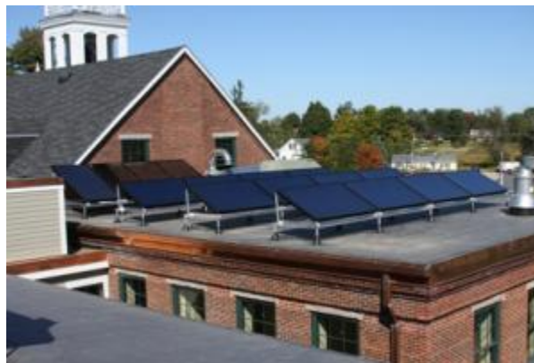
Figure 5. Photo of a Commercial Solar Heating System on a Roof
