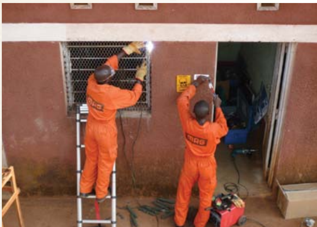
The physical security team improves the security of a police armorer's window.
