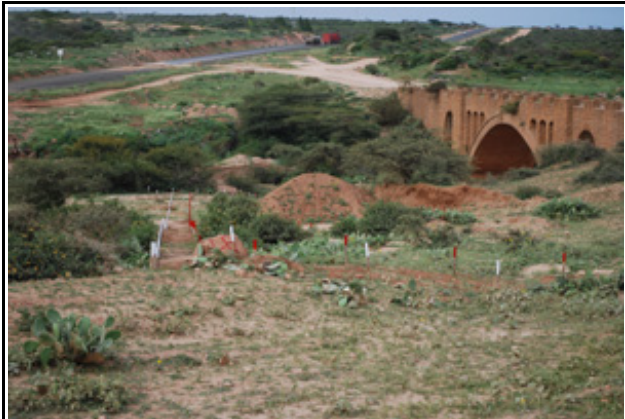
EMAO Technical Survey in support of highway construction.
