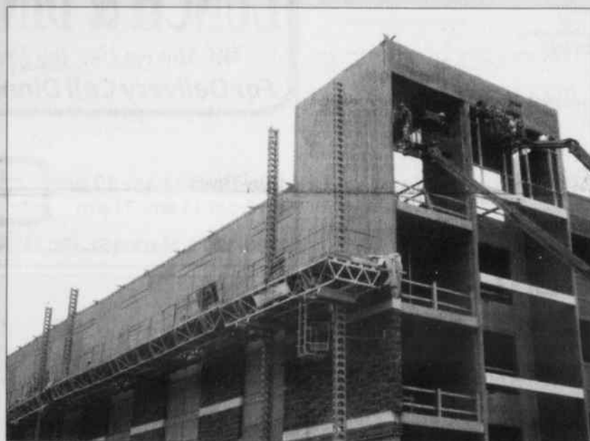
Construction workers continue to erect the new parking deck on South Main Street.
