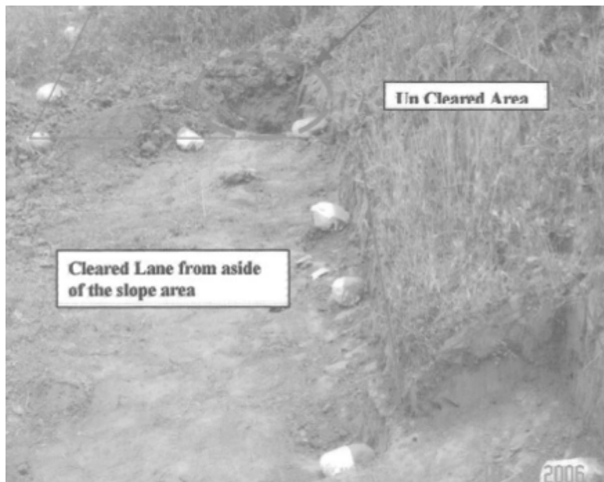
“Cleared Lane from aside of the slope area”
