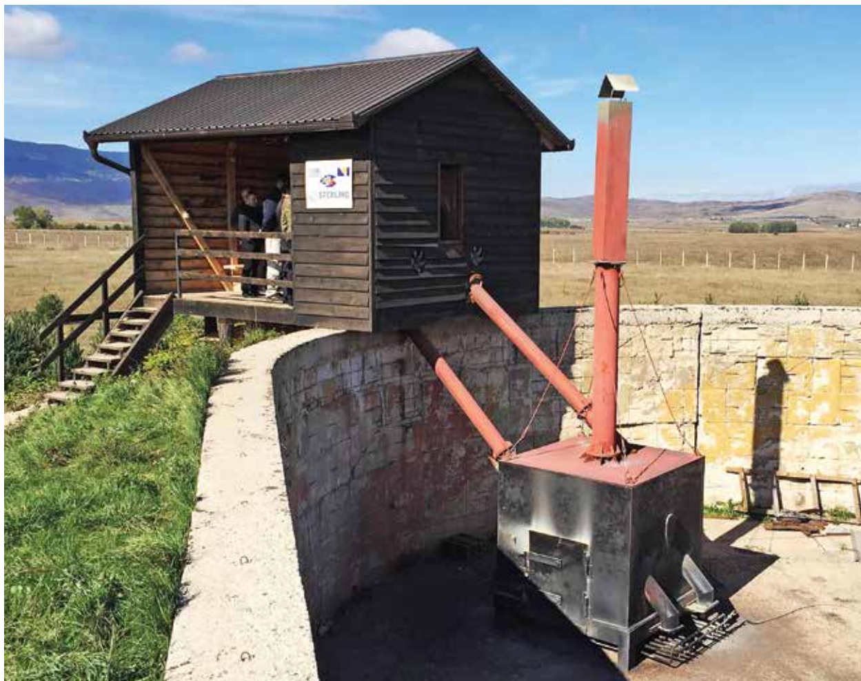
Personnel load items into the furnace via one of two chutes. Gas burners below furnace raise internal temperature above 250 degrees Celsius (482 degrees Fahrenheit).
