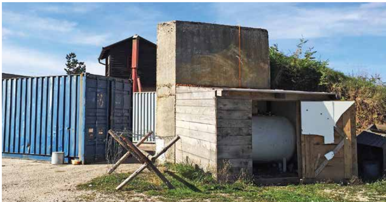
Earth, concrete and steel containers form a concave barrier away from personnel in the chute structure.
