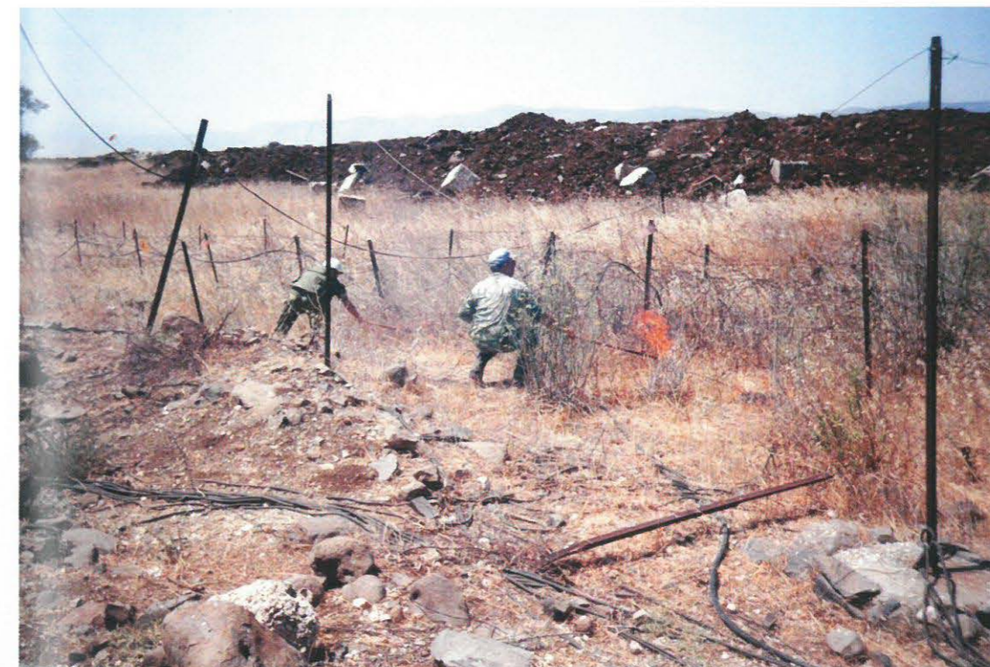
Engineers prepare to burn vegetation in a suspected area to make clearance easier and expose trip wire threats.
