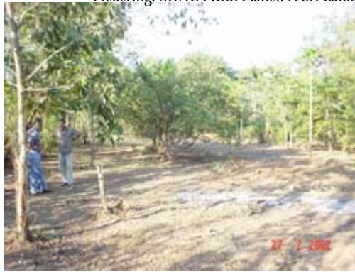
Clearing an area for MFP's MDD Training & Assessment Centre in Sigriya, Sri Lanka.
