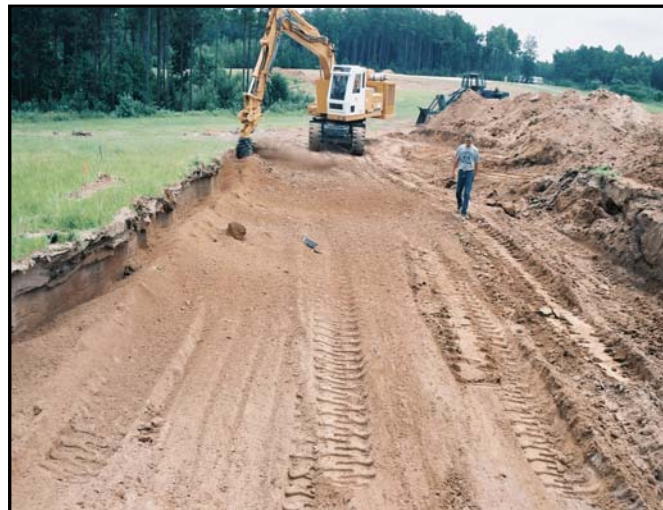
Figure 12. Vertical Mill Completing a Rearward Pass
