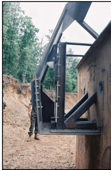
Figure 20. Witness Plates After Second Blast
