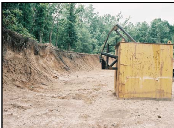
Figure 14. Shield Before Blast
