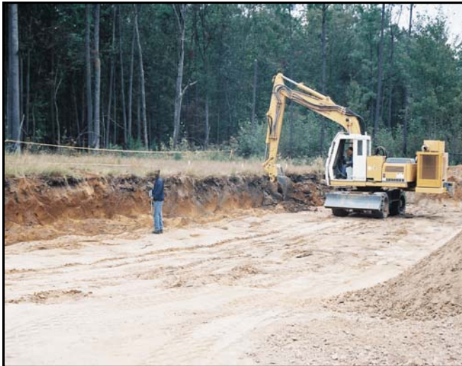
Figure 22. Blind Test - Excavation
