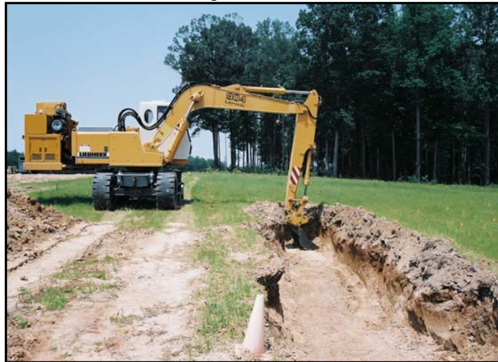
Figure 7. Working Across Trench
