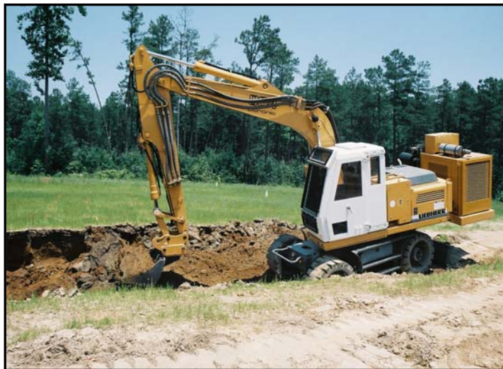
Figure 8. Working Inside Trench
