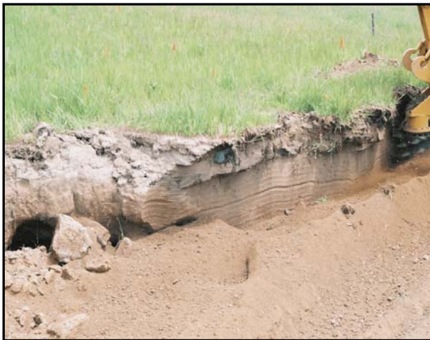
Figure 11. Mine Exposed in Bank with Vertical Mill
