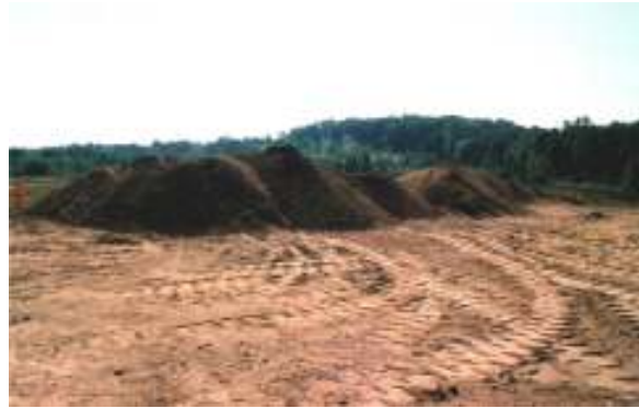
Figure 11. The Sifted Soil From the Test Site 1 Berm
