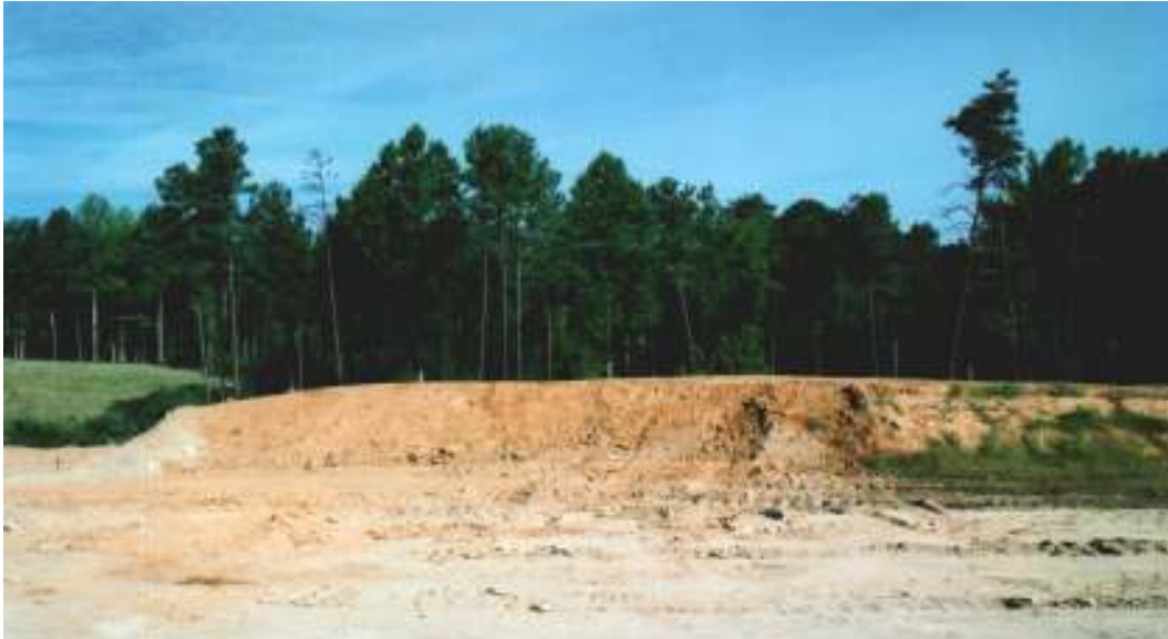
Figure 8. Berm at Test Site 2
