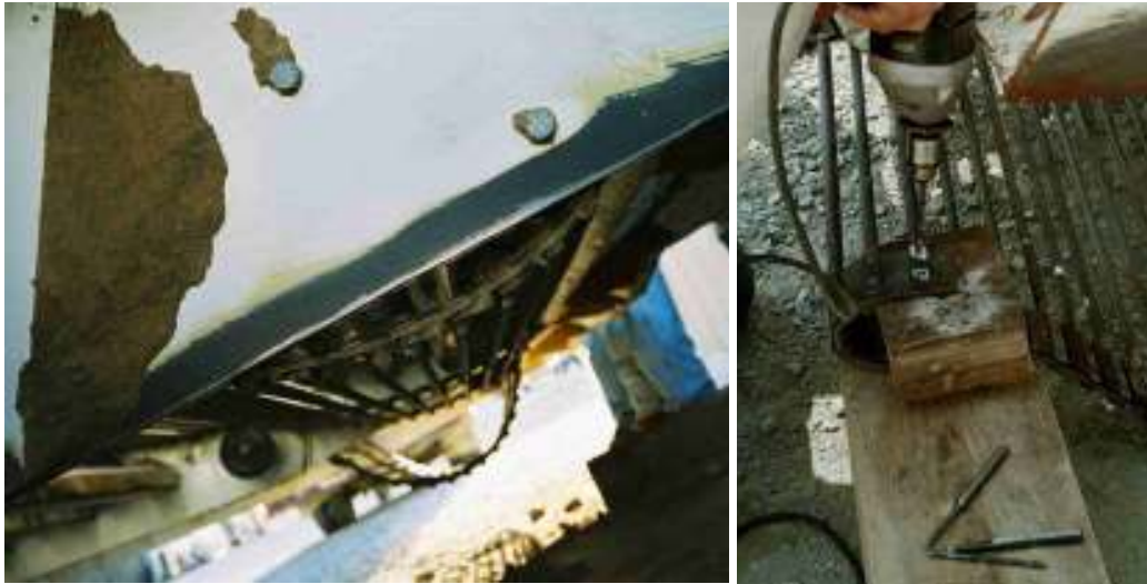
Figure 24: Loose MCS Belt Repair
