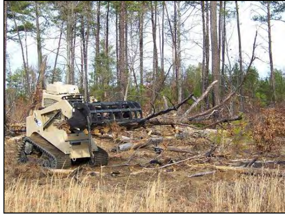
Figure 32: Removing Branches and Other Vegetation Debris
