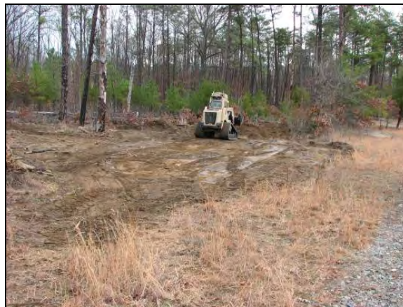
Figure 38: Grading with the 4-in-1 Bucket
