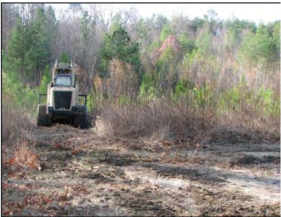
Figure 25: Category 1 Vegetation, Before Cutting
