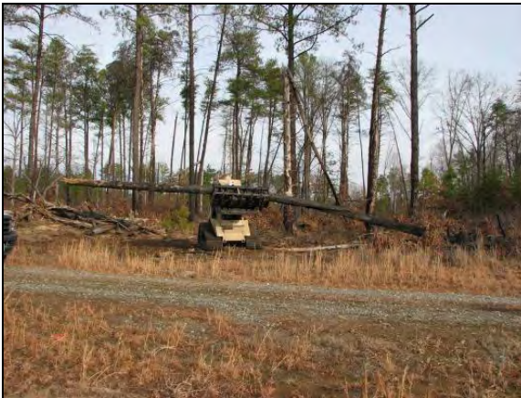
Figure 33: Removing Large Tree
