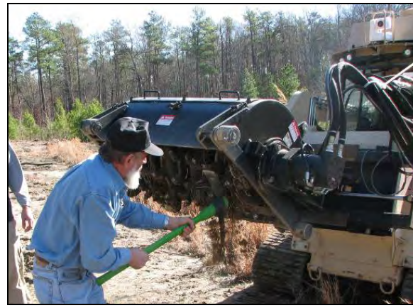
Figure 54: Removal of Dirt and Vegetation Accumulation
