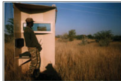
Protective Blast Shield.
