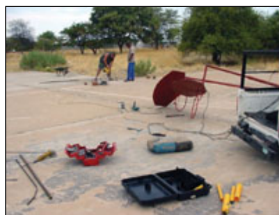
Basketball court construction.
