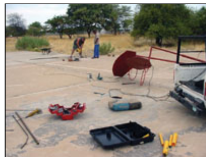
Basketball court construction.
