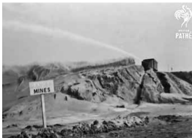
Figure 9. Royal Engineers make use of water jets while clearing Saunton Sands in Devon, 1947. 21 Figure courtesy of British Pathe.
