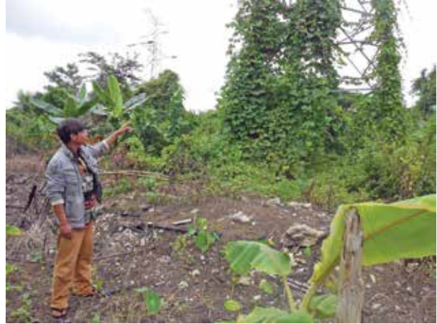
A key informant shows the hazardous area around an electricity pylon. No fences or signs warn the local population, Pa Ra Hi Ta village, Loikaw township, Kayah State.
