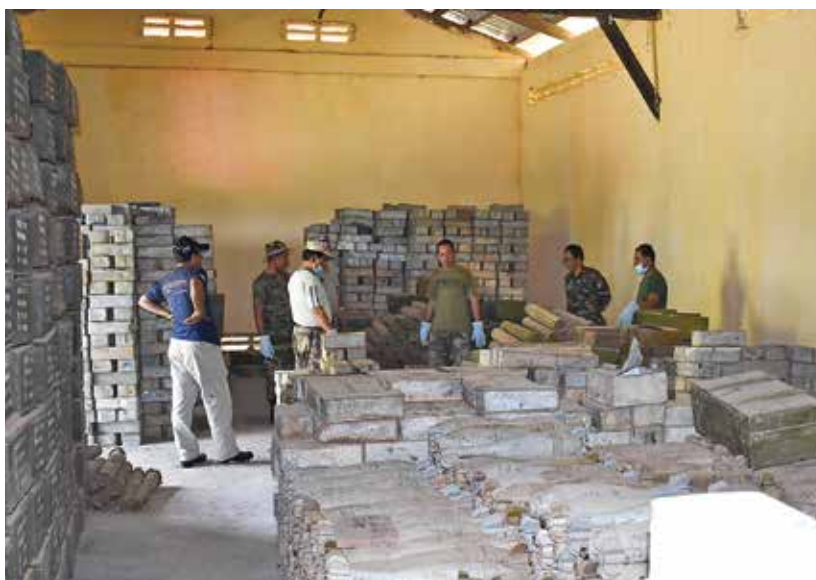
Typical storage conditions before reorganization within the Explosive Store House (ESH). All photos courtesy of Golden West Humanitarian Foundation.
