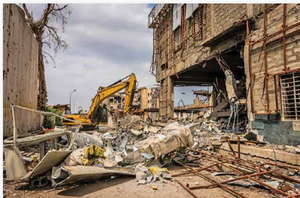
Al-Shifa Hospital: armored heavy equipment operations. Image courtesy of United Nations Mine Action Service Iraq/George Tan.
