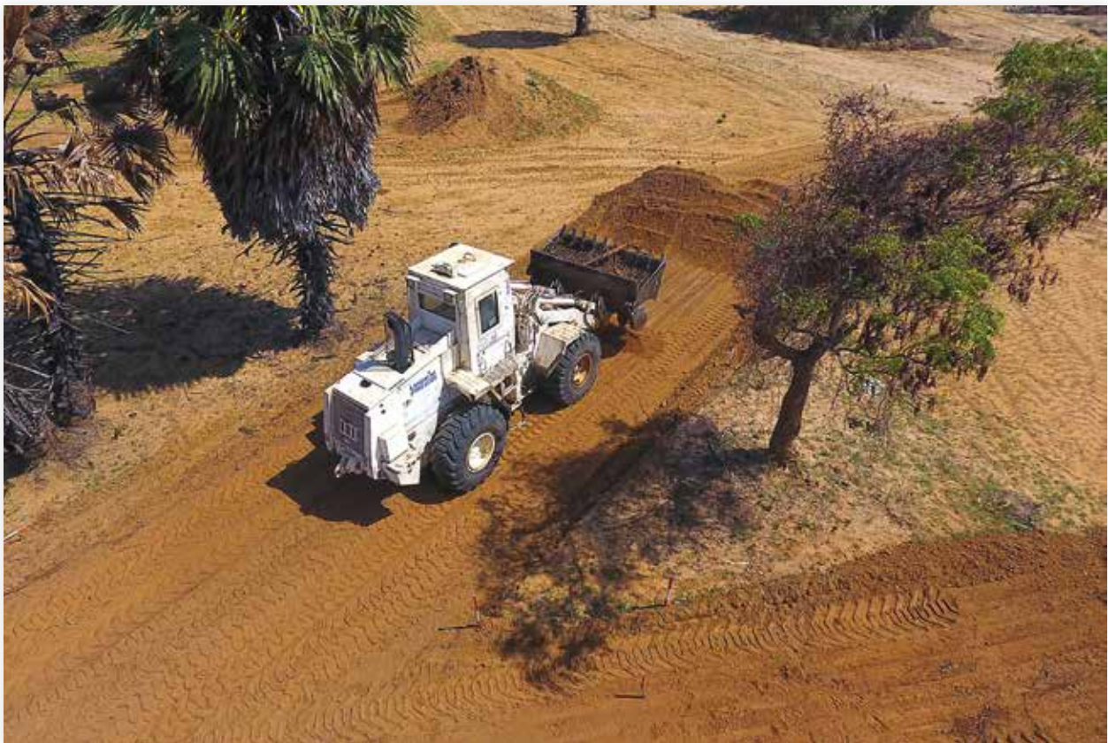
A Case 721C Wheel Loader drops contaminated soil in a marked inspection lane. Aerial photos enable proactive deployment into areas that are best suited for certain assets. Images courtesy of The HALO Trust.
