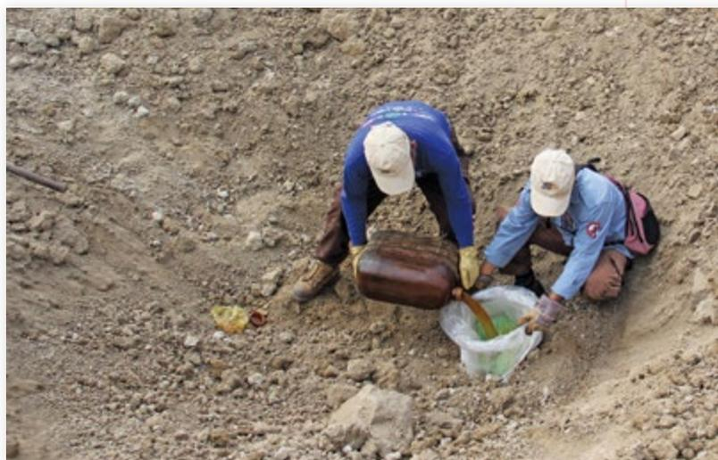
Two of Austin's assistants pour liquid explosives into a bag containing 1,000 U.S.-made 20 mm HE projectiles. This method, which Austin explained, significantly reduces the chances of "kick-outs" during demolition operations. After completing the shot, all participants searched for kick-outs, and none were found.
