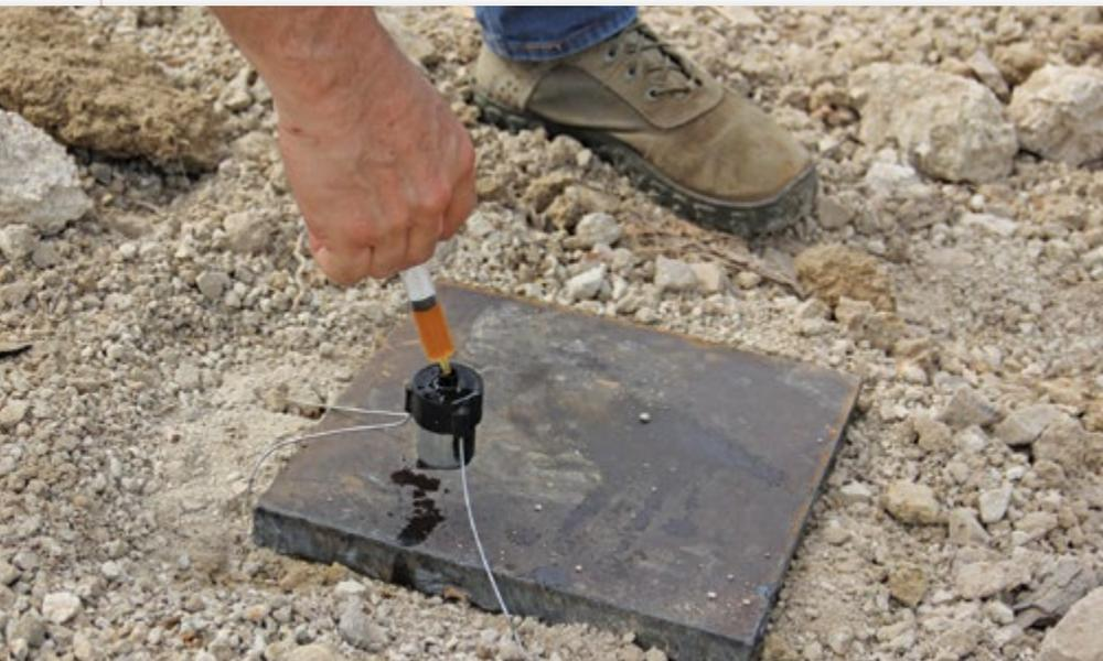
Austin from Golden West fills a shaped charge container with 35 ml of NMD liquid explosive
