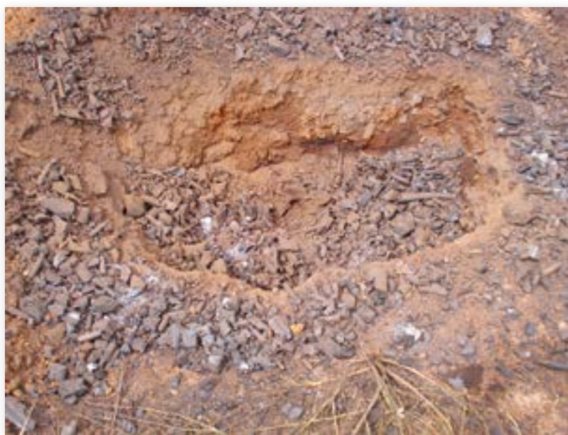
An SAA burn pit. The SAA was burnt in an open pit with a simple metal cover. The slag residue was subsequently buried. This method is hopefully no longer used by operators. Burying the slag residue from SAA pit burns concentrates the toxic waste and is potentially a significant pollution risk. Image © Private.
