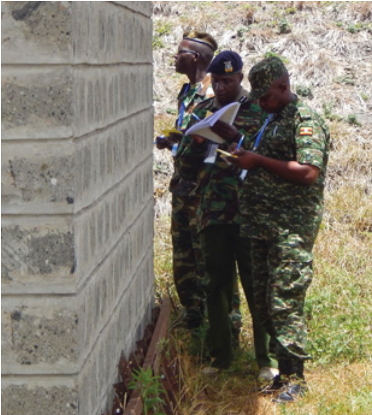
Figure 6. A group of regional PSSM course participants assessing the outside security parameters of an ammunition storage facility during a practical exercise.
