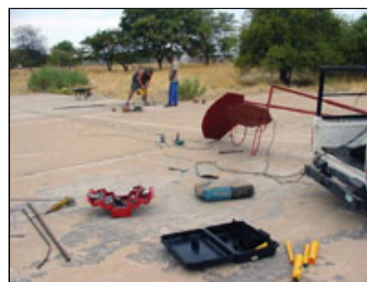
Basketball court construction.
