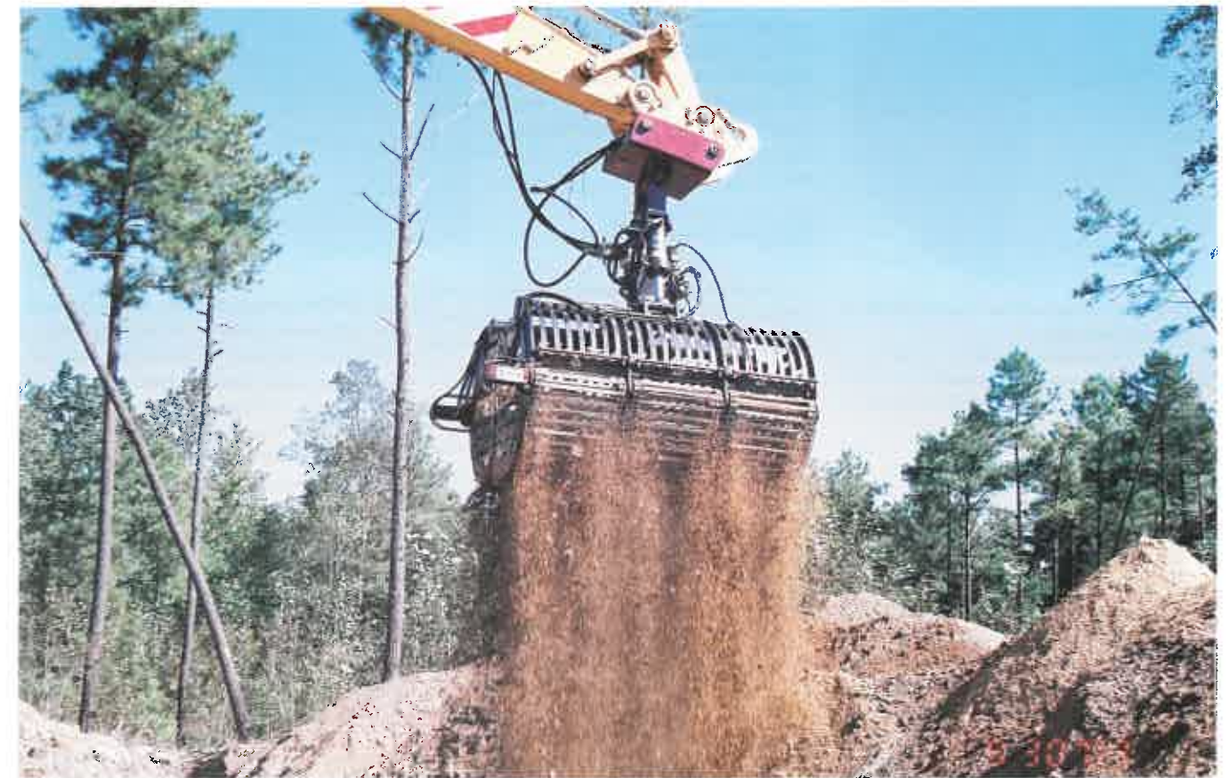
Sifting/Backfilling trench.
