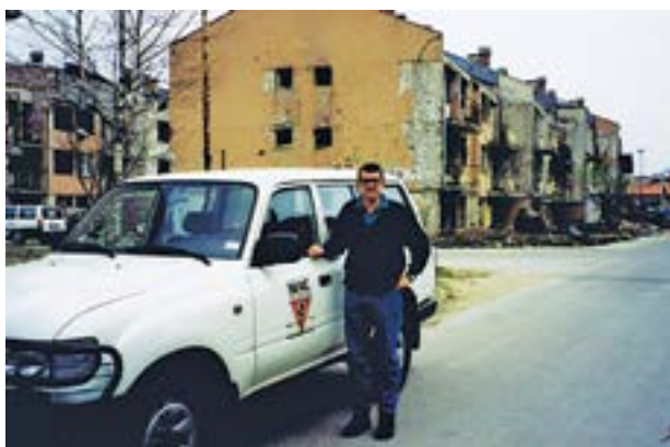
Ian Mansfield stands in front of damaged apartments in Sarajevo. Photo courtesy of the author.
